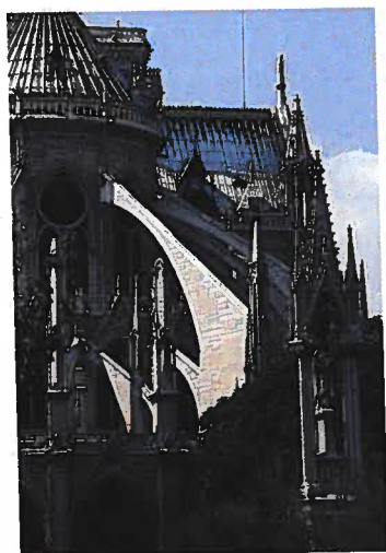
FIGURE 9-34 Flying buttresses (on the cathedral of Notre Dame, in Paris).
