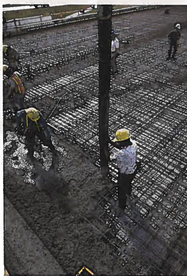
FIGURE 9-29 Steel rods waiting for concrete to be poured around them to form a new highway.
