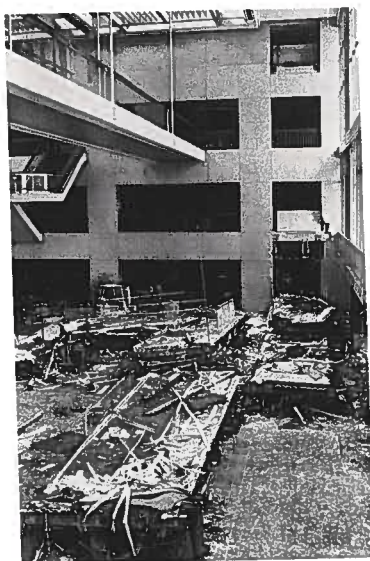
FIGURE 9-2 Elevated walkway collapse in a Kansas City hotel in 1981. How a simple physics calculation could have prevented the tragic loss of 100 lives is considered in Example 9-14.
