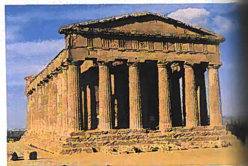
FIGURE 9-23 This Greek temple, in Agrigento, Sicily, built 2500 years ago, shows the post-and-beam construction.
