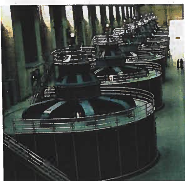
FIGURE 21-15 Water-driven generators at the base of Boulder Dam, Nevada.
